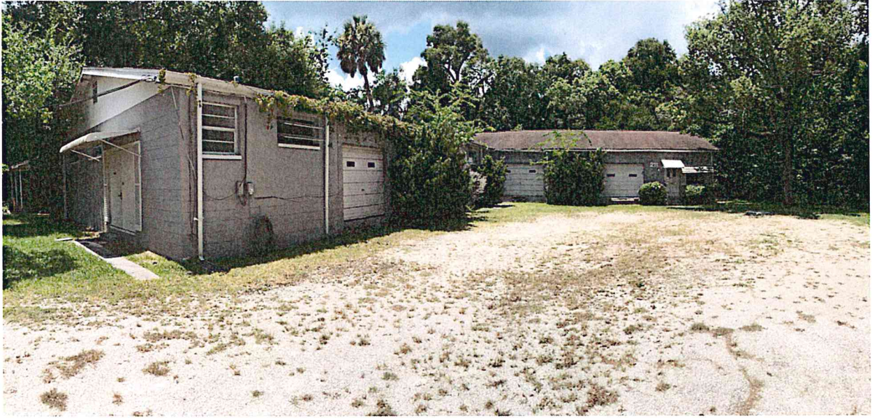
Property Before Façade Grant
